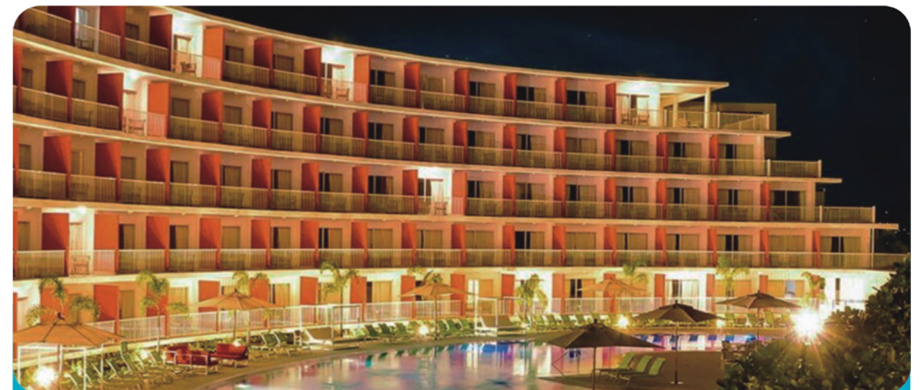
Montego bay resort in Jamaica, with DC inverter VRF system.
