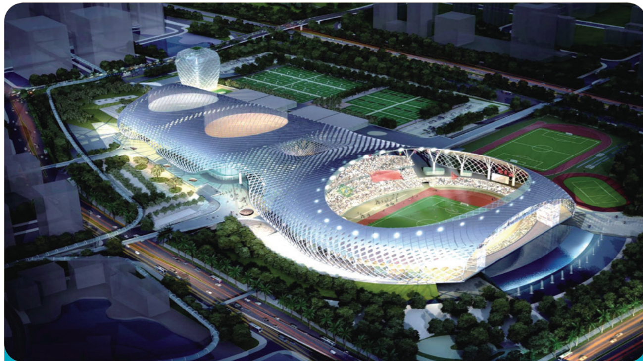
Main venue of the Universiade in Shenzhen, total VRF capacity 8000kW.
