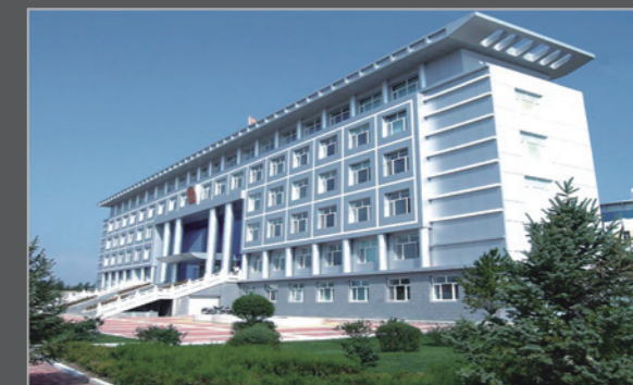
Government building in Inner Mongolia, China.
